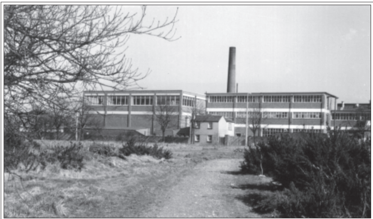
'The Creameries' site from 'Workhouse Path', c.1966. The old Workhouse Master's Lodge is centre foreground. (Photograph reproduced by courtesy of Eric Montague)
