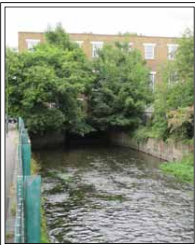
Connolly's Cut leading to Connolly's Mill
