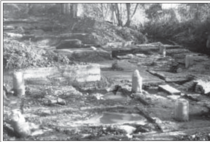
The concrete foundation pillars of the former CITB workshops protruding through those of Bennett's mill. (D Luff)
