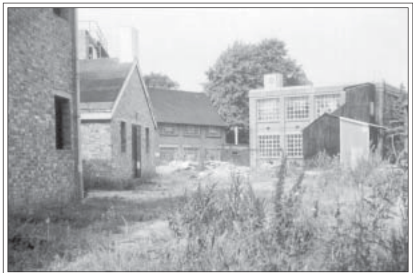
To the left, two of the CITB workshops on the Bennett's site, c.1980 (D Luff)
