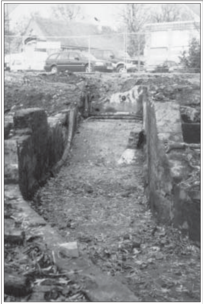
The former waterwheel channel from Bennett's mill, that had been buried since 1974. Looking south to Bennett's ditch (D Luff)
