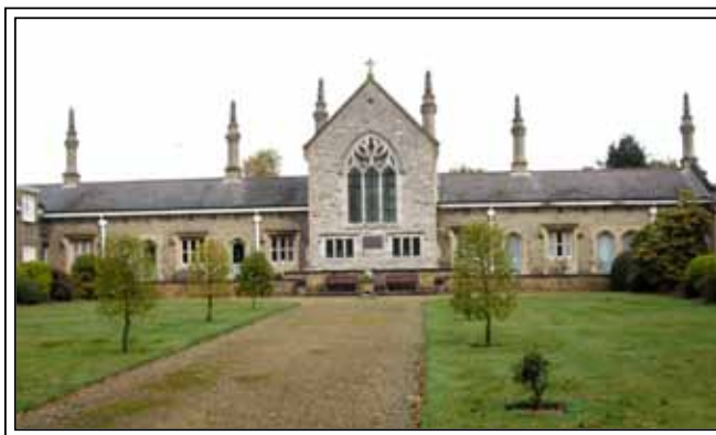
The central wing of the Leathersellers' almshouse in Barnet. Photo October 2012 JG
