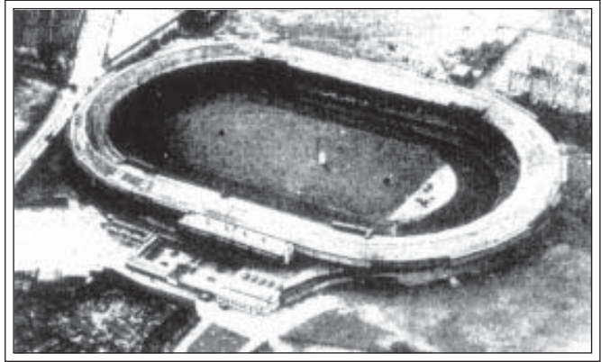
Wimbledon Stadium, shortly after opening (Wimbledon Boro' News 9 March 1934)
