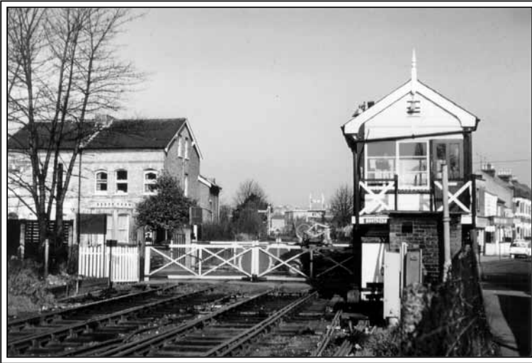
Merton Park signal box and level crossing on the Kingston Road in 1977 D Luff
