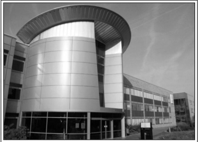
Recent building at South Thames College Morden campus. Photo: D Roe (2011)
