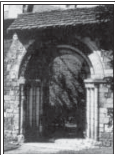
5 Norman Arch re-constructed at Merton Parish Church
