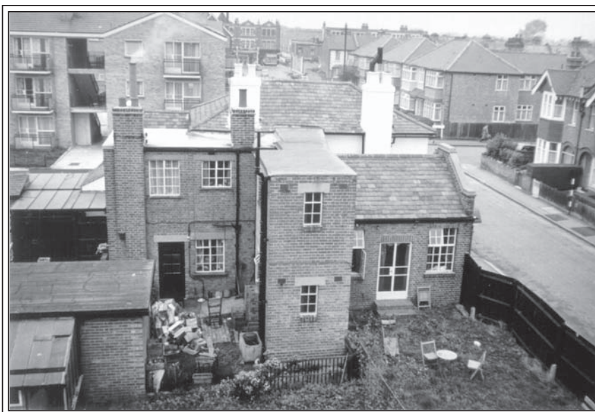
Rear of the Princess Royal , Abbey Road, Merton 1963, photograph by Bill Rudd
