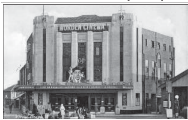
Morden Cinema in 1933, reproduced by courtesy of Merton Library & Heritage Service
