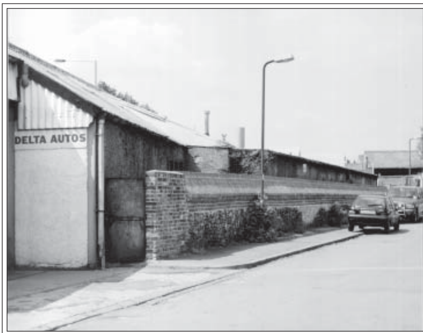
The priory wall in Station Road, after repair. Photo: D Luff
