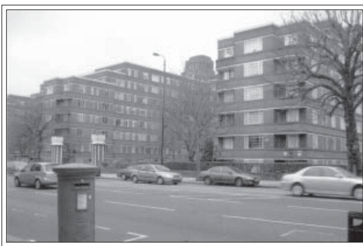
(Part of) Du Cane Court, Balham High Road Photo: JG Jan 2010
